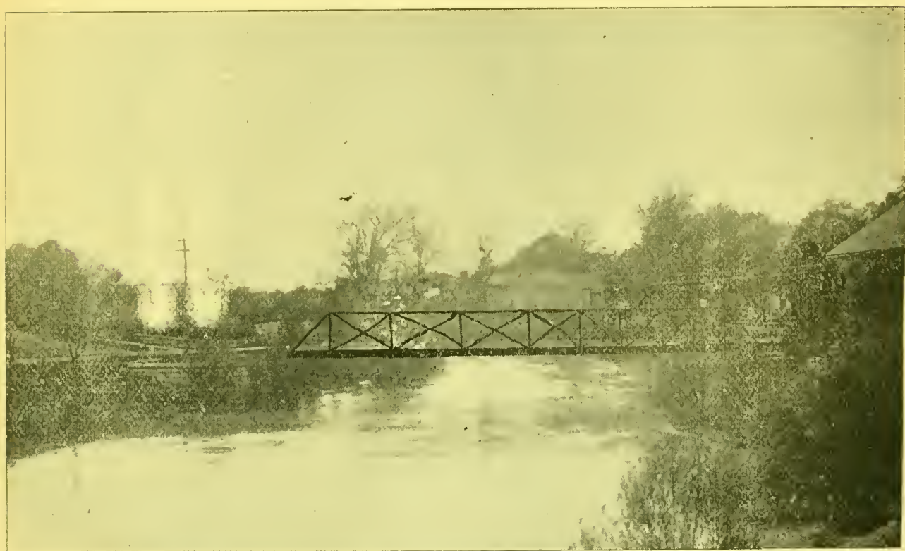
THE TONAWANDA BRIDGE—LAND OFFICE IN THE DISTANCE.
